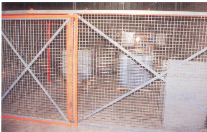
Because of the risks to human health, the tanks with liquid enzymes are stored behind a fence in a secured area.
