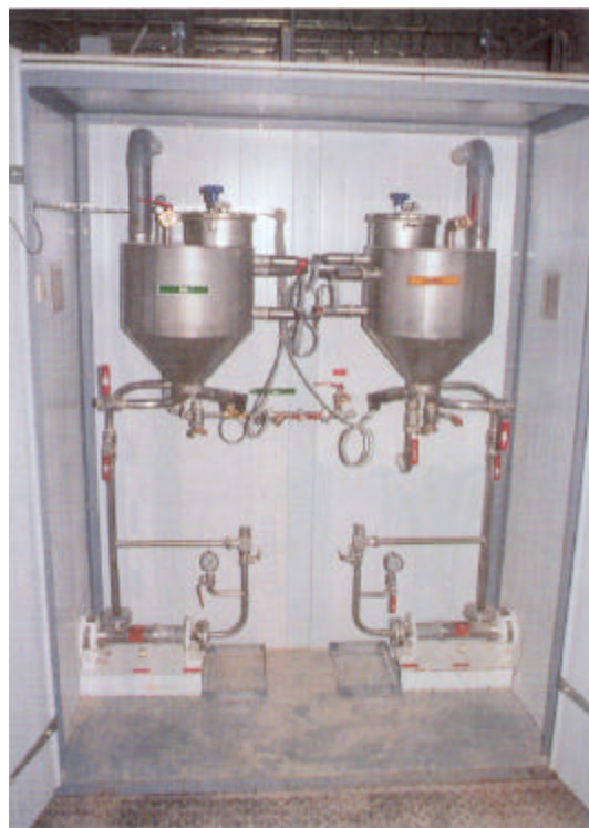
From the large container the enzyme is pumped to this buffer unit (left tank with green sticker). The other unit contains water to dilute the liquid enzymes before spraying.
